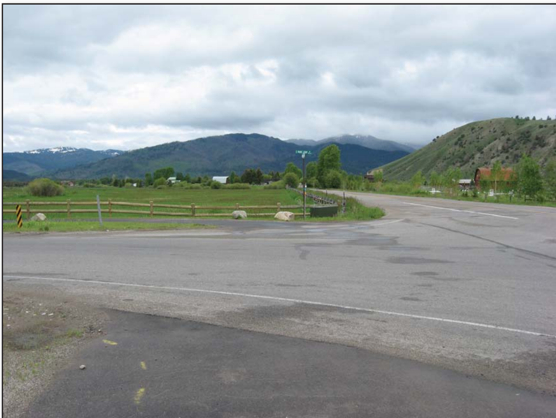
18. South Park Loop Road, view west at Boyle Hill Road crossing
