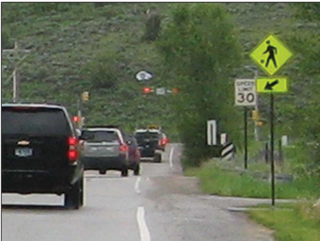
8. High School Road, view east, inconsistent speed limit sign
