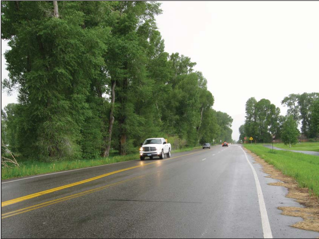
9. High School Road, view east, left turn lane, shoulders
