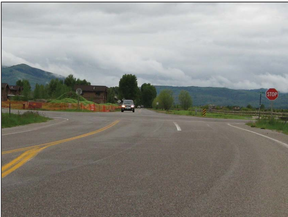
14. Tribal Trail Road, view south, through-lane off-set
