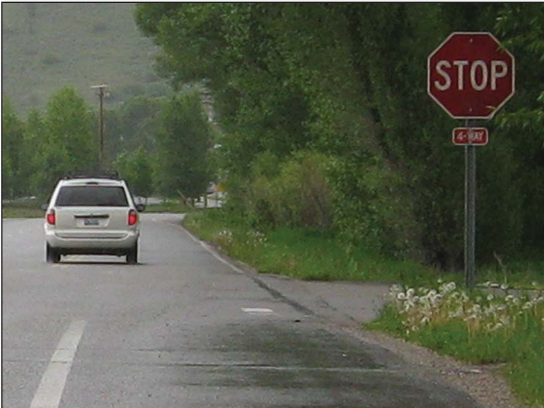
10. High School Road, view east, through-lane off-set
